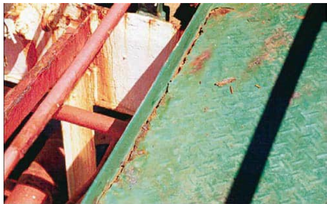
Catwalk cracked.
